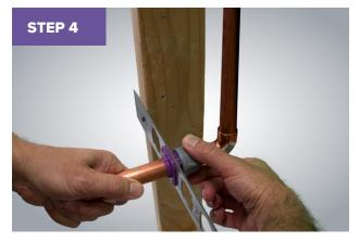
Slide a 3/4" tube or bullet through the insert. Lock the tubing in position by tightening the grey nut clockwise, by hand.
